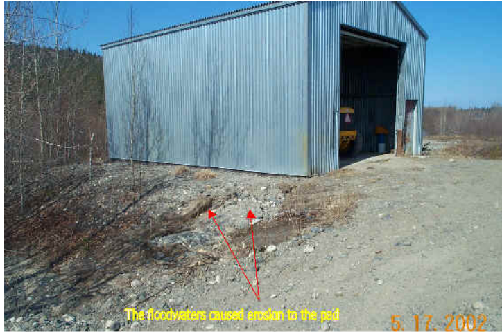
Photo 1: Airport maintenance shop building pad erosion, May 17, 2002.
