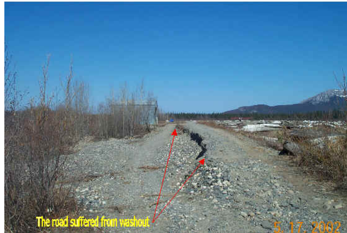
Photo 3: The airport access road erosion damage, May 17, 2002.
