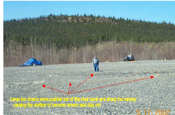
Photo 2: During the spring break up 2002 flood, large chunks of ice caused erosion of the gravel airport surface, May 17, 2002.
